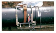
6. Connection of 40 V standard automatic welding machine for electrofusion sockets to existing 4 mm contacts.
