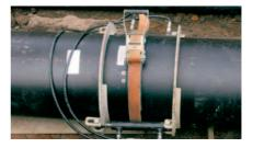
Attachment of tensioning tool (in this case a strap) to reduce the joint width and exert required pressure for joining.
