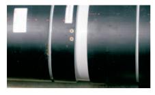
Insertion of spigot end into socket on a carefully prepared, clean surface.
