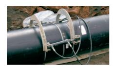
Adjustment of hydraulic clamping device.
