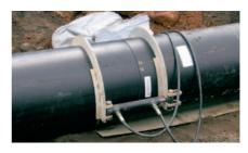
4. The two pipe ends are brought together by means of hydraulic force.
