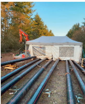
Top: installation of pipes using the horizontal directional drilling method (HDD). Bottom left: parallel welding in a tent of several cable protection pipe strings in the heating element butt welding process. Bottom right: SIMONA® PE 100 cable protection pipes delivered to the Moselle slopes near Bullay.
