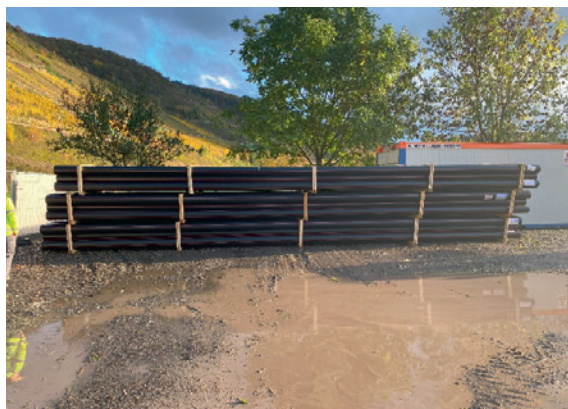
Top: installation of pipes using the horizontal directional drilling method (HDD). Bottom left: parallel welding in a tent of several cable protection pipe strings in the heating element butt welding process. Bottom right: SIMONA® PE 100 cable protection pipes delivered to the Moselle slopes near Bullay.
