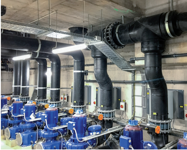
Left: SIMONA® PE 100 pipelines, PE 100 tees with reduced outlet and PE 100 stub flanges were used for the bathing water treatment plant. Right: The Captura® filtration systems from aquila were made with SIMONA® PP-H AlphaPlus® sheets.
