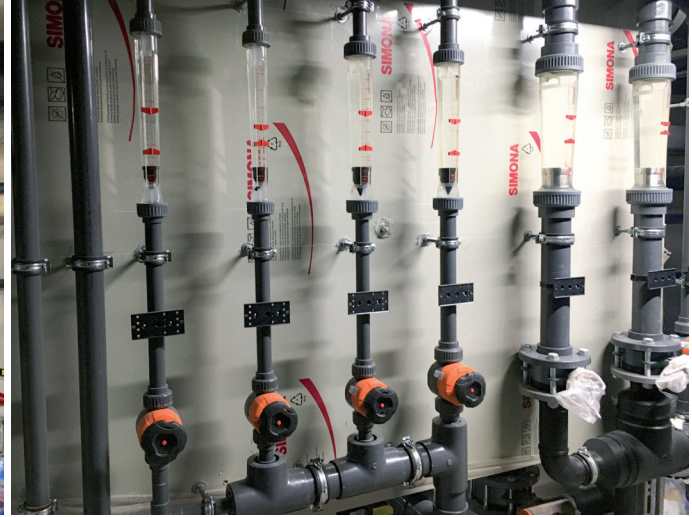
Left: SIMONA® PE 100 pipelines, PE 100 tees with reduced outlet and PE 100 stub flanges were used for the bathing water treatment plant. Right: The Captura® filtration systems from aquila were made with SIMONA® PP-H AlphaPlus® sheets.
