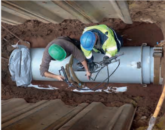
Open-trench pipe laying with sand bed and trench boxes (PE 100 grey/UV-stabilised; d 710, SDR 17.6)
