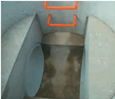
View of concrete shaft with SIMONA® PE Shaft Connection SIMOFUSE® Type C
